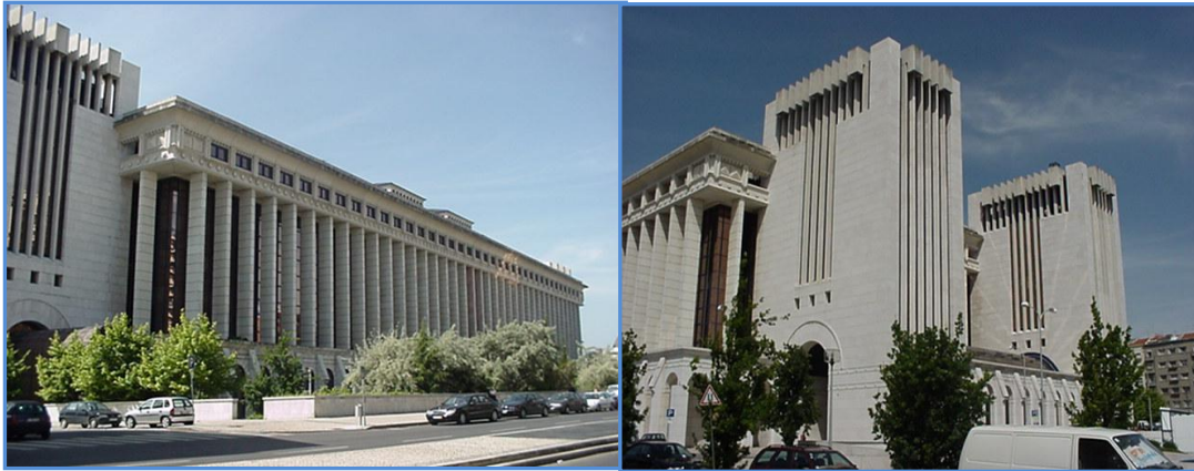
Figures 2.1 and 2.2- Caixa Geral de Depósitos central and East Blocks
